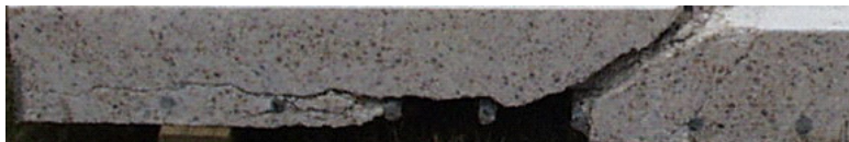
c) Crack Pattern at Ultimate Load from Experiment
